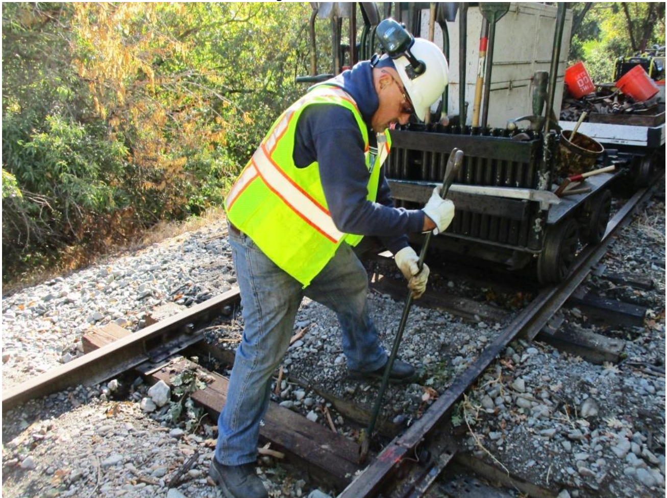
Dave W. pulls on a track-wrench to get the nuts off the bolts holding the wonky joint together
