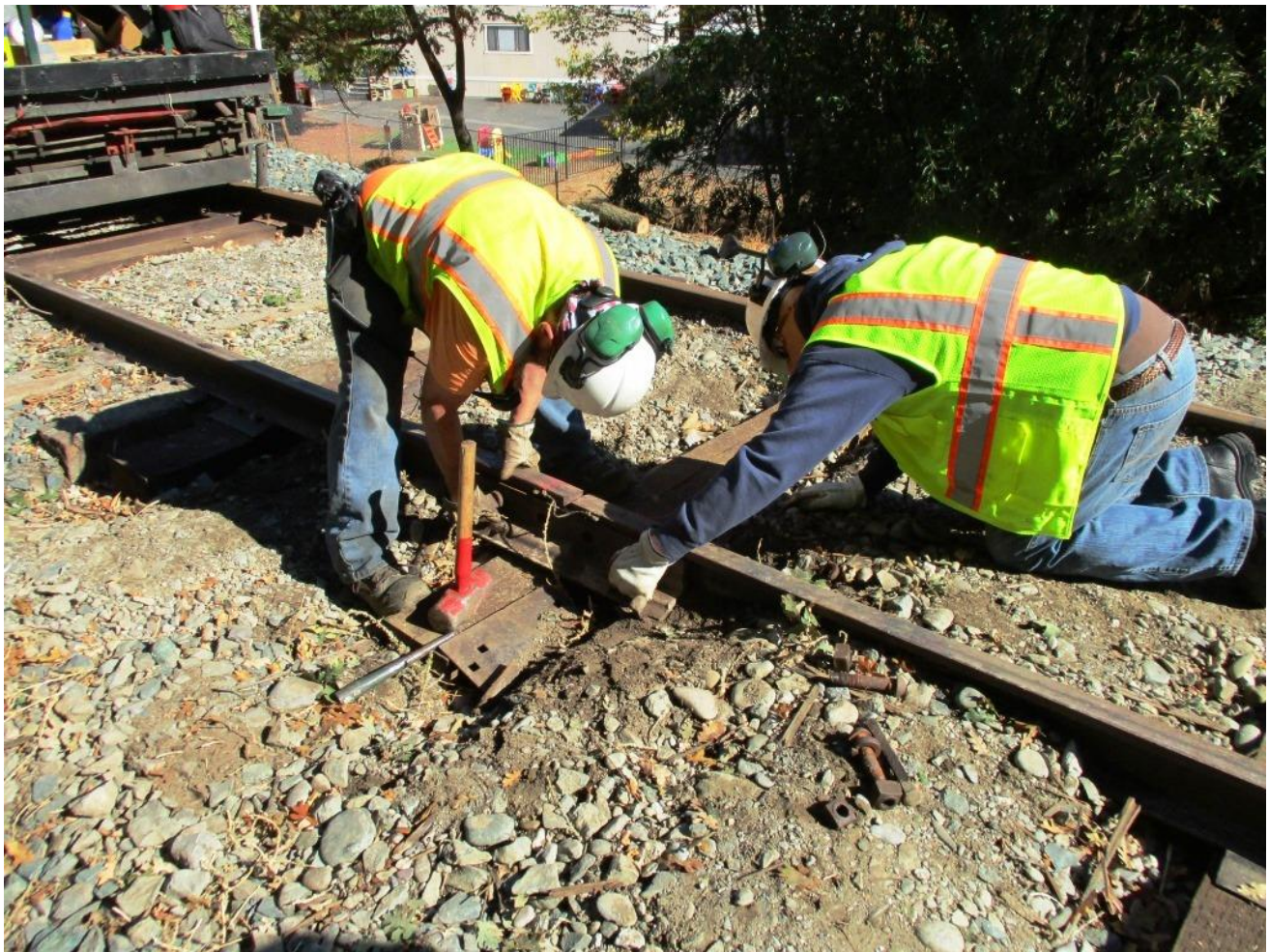
Joe and Dave W. get the joint-bars reattached to the rail
