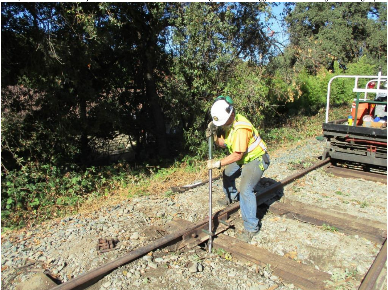
Joe gets the rail to shift into position to be bolted up again
