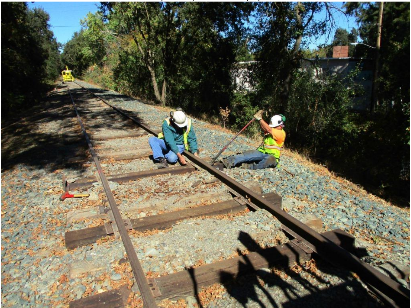
Joe nips up the rail for Alan to insert a tie-plate
