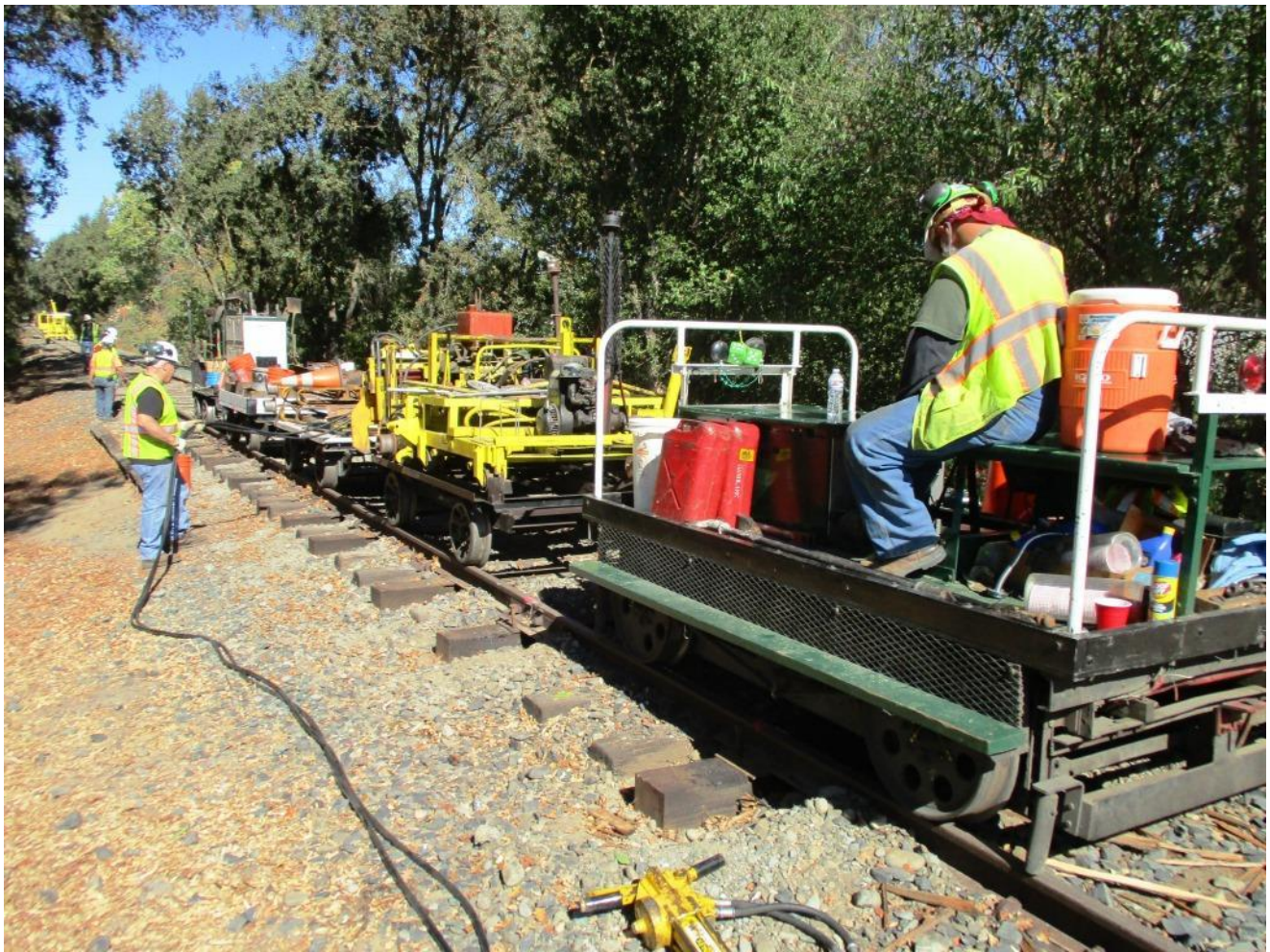
The hydraulic spike-driver is deployed
