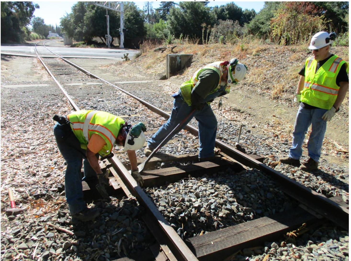
Mike F. nips-up the rail as Joe gets a tie-plate placed
