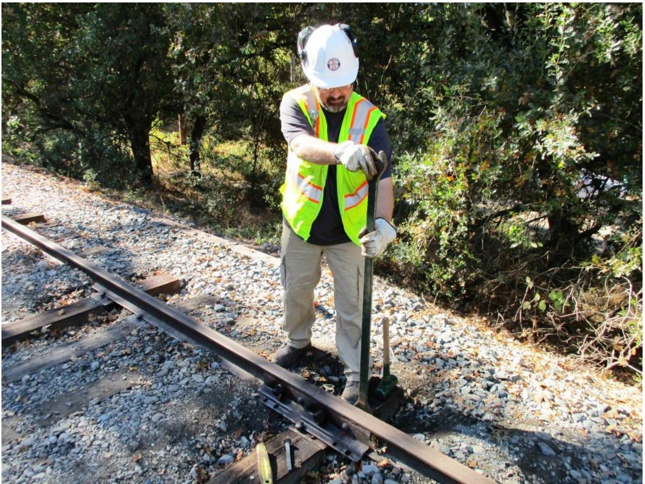
DJ retightens the bolts on the joint immediately to the south
