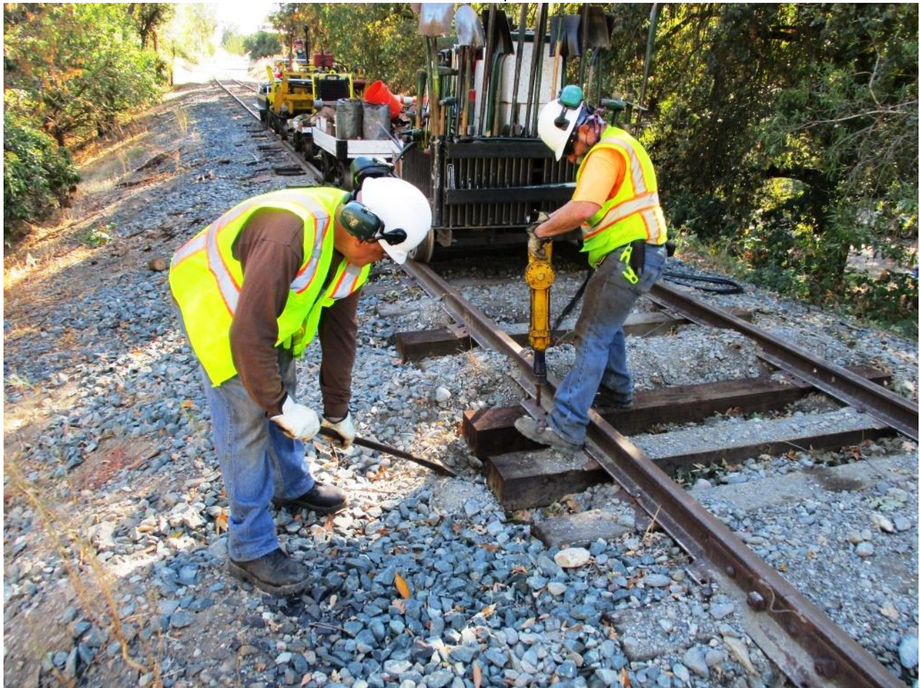
Then Joe takes on the hydraulic spike-driver and Dave W. nips-up the tie
