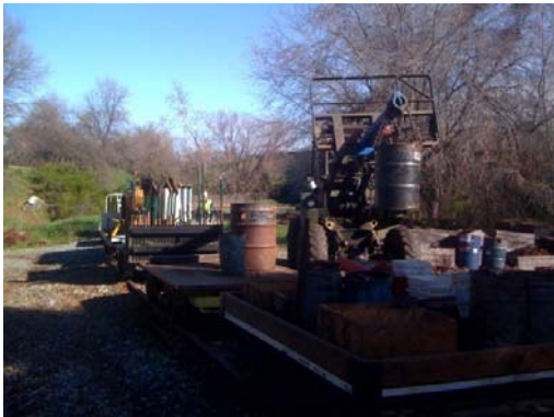
MOW work train being loaded with rail anchors at Setzer yard.
