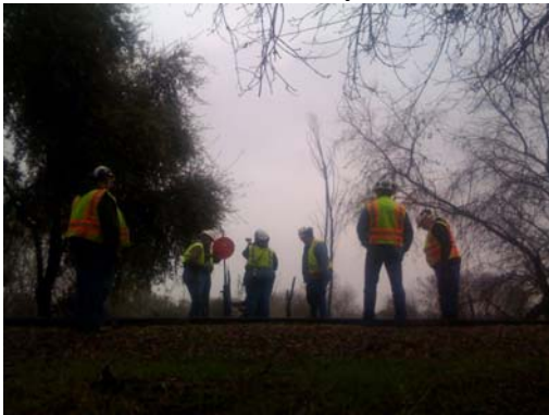
The MOW Crew working on switch #16
