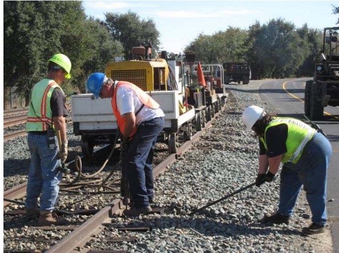
(l-r) Steve, Wolfgang, and Heather spiking down new ties with the spike hammer and air compressor. Steve set the spike, Wolfgang drives the spike and Heather nips the tie.
