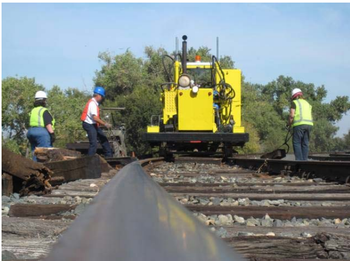
(l-r) Heather, Wolfgang, and Janet all working with the Tie Shear cutting ties along the SSRR Mainline at Baths.
