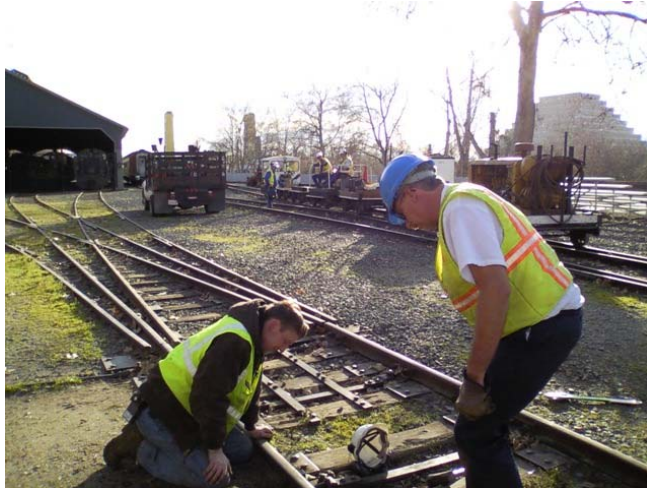
Richard and Wolfgang work on Switch #3 in the Old Sac. yard.
