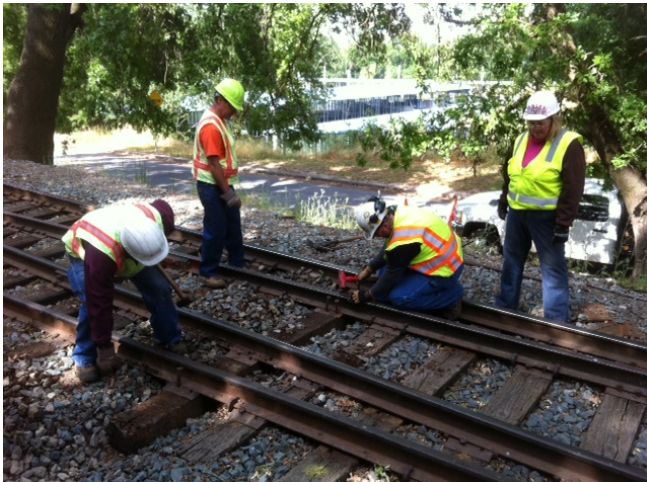
(l-r) Jon, Steve, Mike, and Janet set spikes in a newly inserted tie on switch #14
