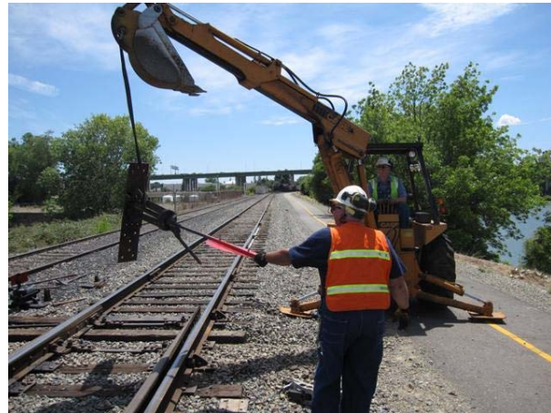
Chris and Harry using the backhoe to remove the switch stand at Clunie on Saturday.
