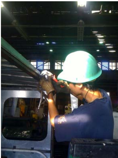
Bert working on the motor car roof. Almost Done!
