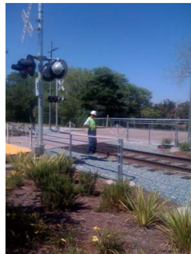
Clem out on the mainline while servicing switches.
