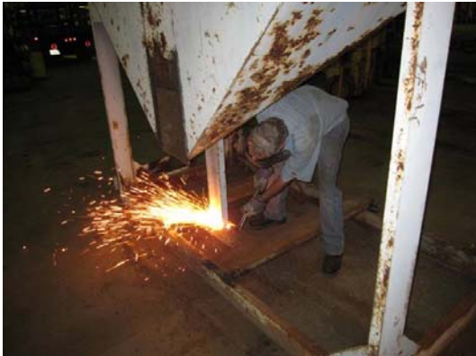
Jim converting the side dump bin to a center dump bin
