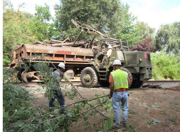
Mike on the Green Machine loading the side dump car with dead ties while Brenton and Jack clear away limbs from a fallen tree.
