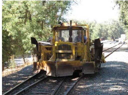
Ballast Regulator moving onto the mainline
