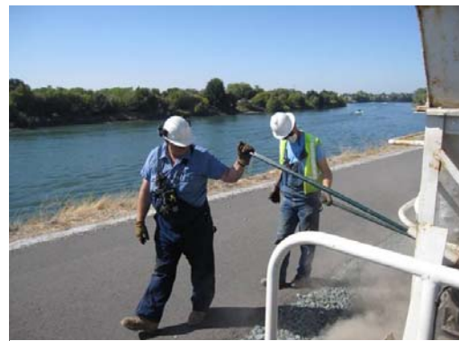
Chris and Steve dumping ballast on Saturday
