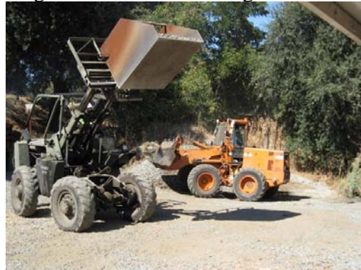
Green Machine and Loader filling the ballast carts
